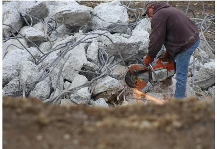
*Cutting rebar in the old spillway
